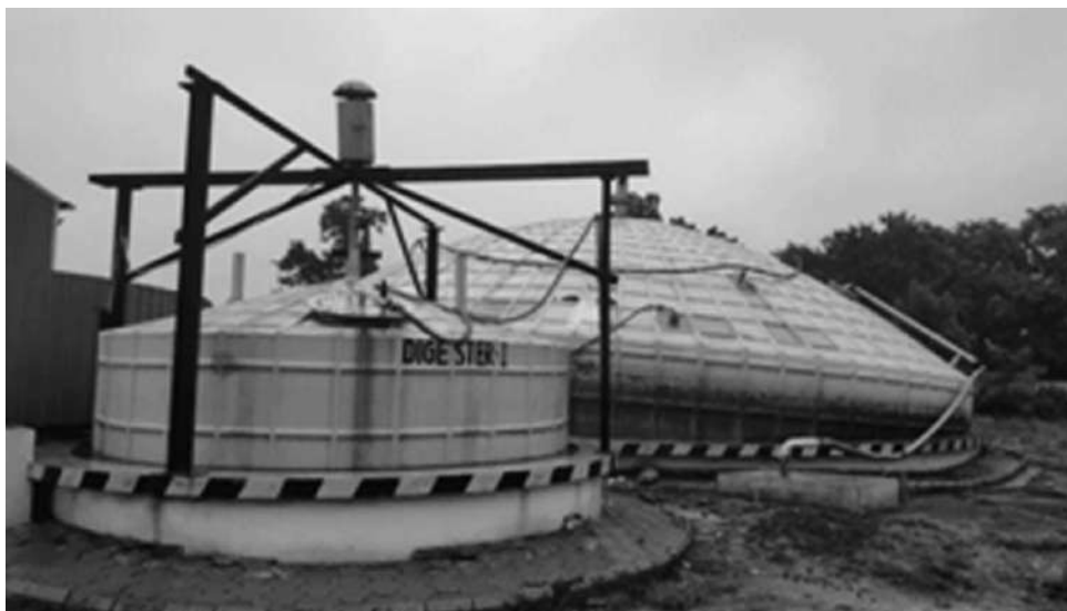
Figure 8: The Biomethanation Facility Opposite the Vegetable and Fruit Market. Organic Waste is Converted to Fuel used by City Buses and as Cooking Fuel
